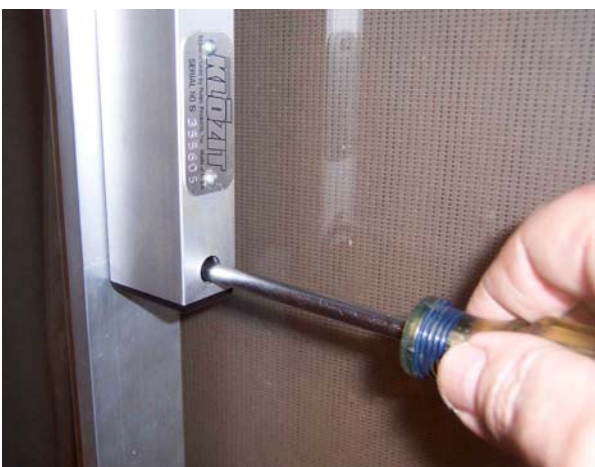
Removing bottom mounting screw
