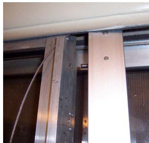
Pulling roll pin out of hole in door frame
